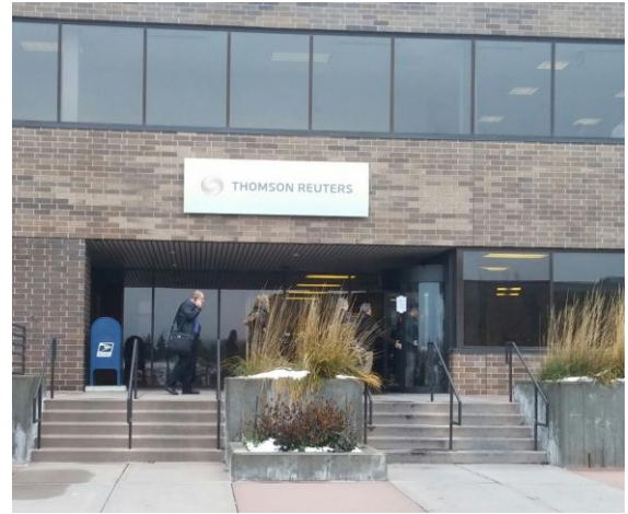
C Building Entrance
