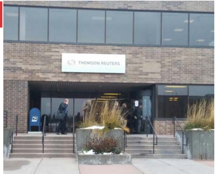
C Building Entrance
